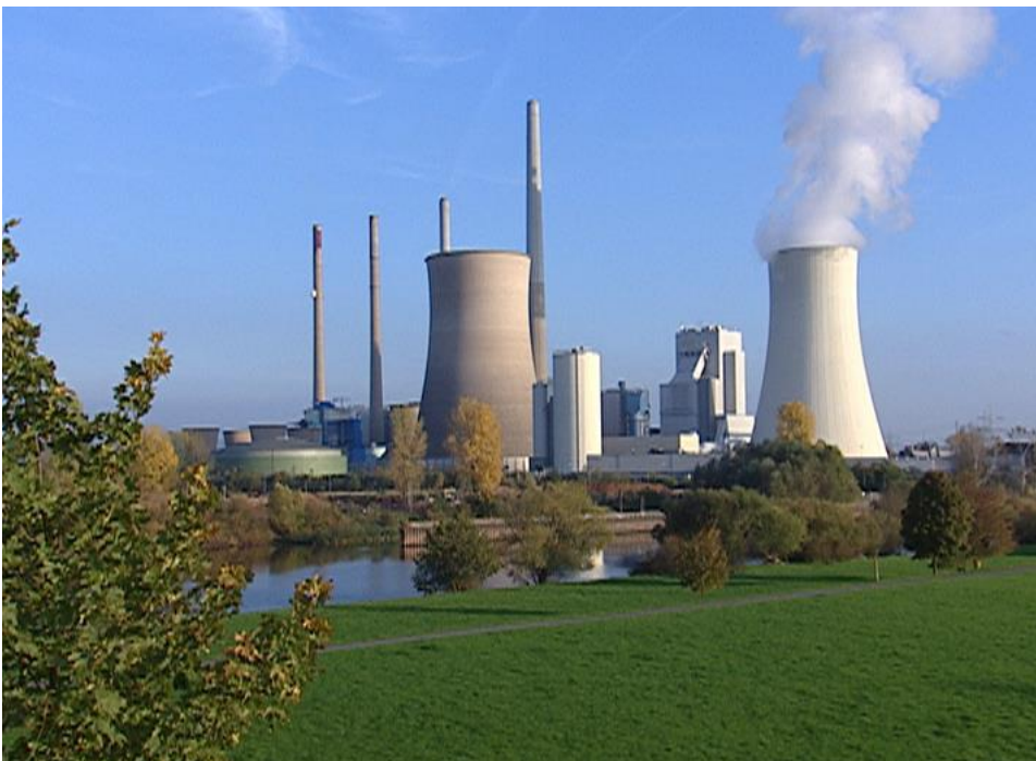
Staudinger Coal-Fired Power Station, E.ON Kraftwerke
